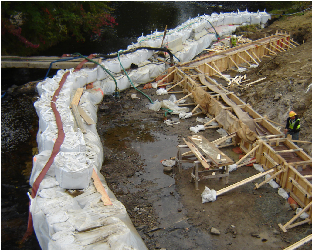
IVI Cubic Yard Bags are an effective solution when used as coffer dams during shoreline construction projects.
